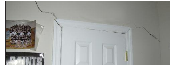
Sometimes things don't work out as planned. Raising and then setting a house is not for the faint of heart and comes with its own set of skill and knowledge requirements. Here, the slightest mishap dropped this house and caused innumerable damage.
