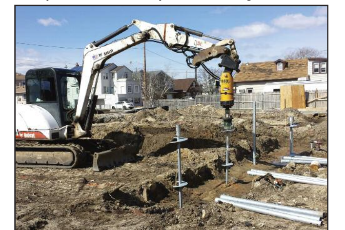
Helical piers (piles) are "screwed" into load-bearing soils. Sections can be extended. Bearing plate(s) are welded to the shaft. Photo courtesy High Rise Industries, Inc.
