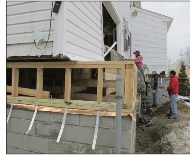
Sometimes things don't work out as planned. Raising and then setting a house is not for the faint of heart and comes with its own set of skill and knowledge requirements. Here, the slightest mishap dropped this house and caused innumerable damage.
